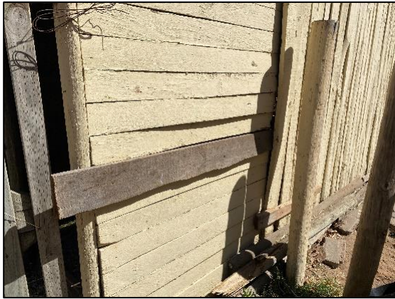
Figure 9. Repairs made to the feed room wall at Tokai stables.
